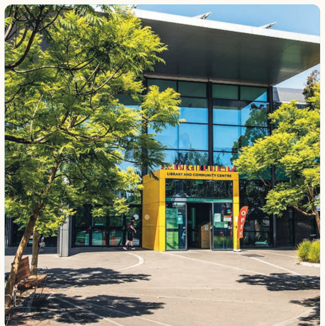
Carnegie Library and Community Centre, Carnegie.
