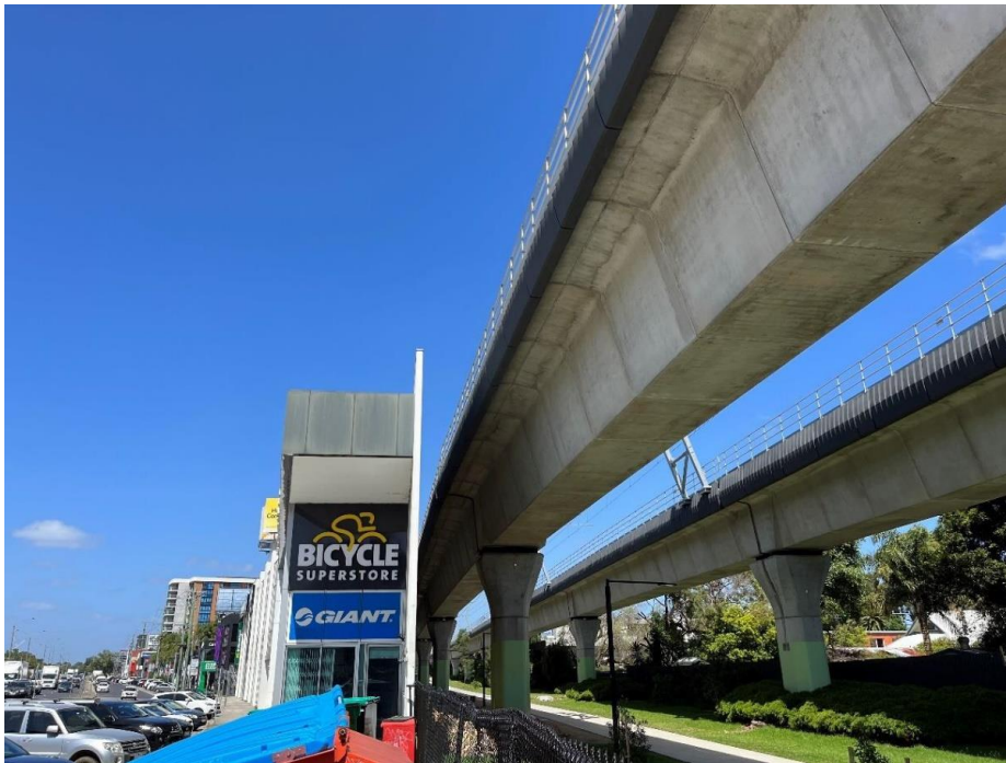
Figure 9 View of 1030 Dandenong Road bound by highway and skyrail
