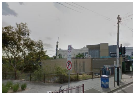
Railway line under Glen Huntly Rd
