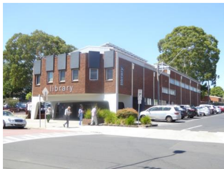
Existing Elsternwick library site and adjoining carparking and access
