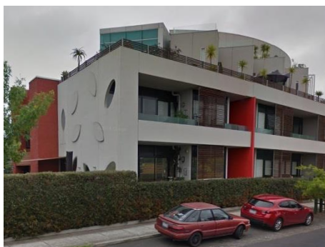
Former police station site on Gordon St
