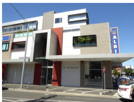
Recent 4 storey development
