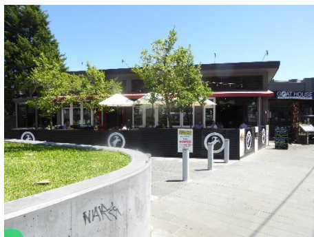
Tenancy fronting Elsternwick Plaza
