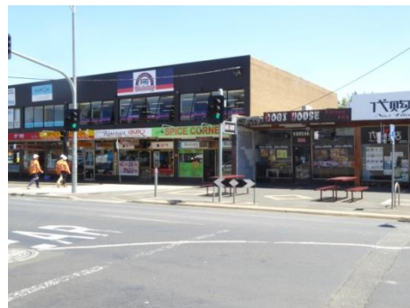
Koornang Road, north of railway line
