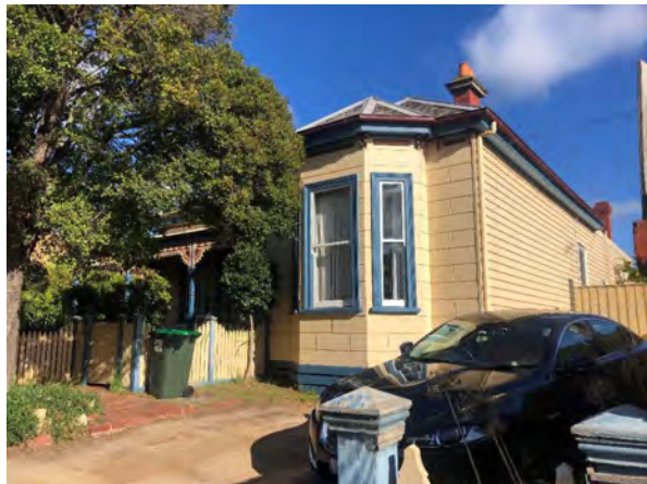
Figure 9. 9 Vickery Street, Bentleigh (Source: GJM Heritage, May 2022)
