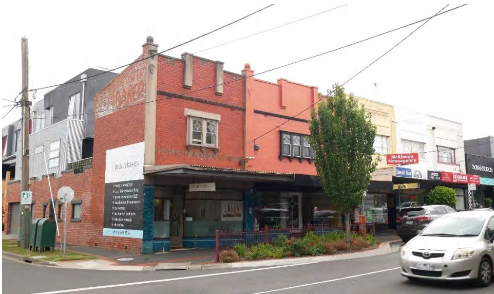
Figure 13. Looking north at 159-167 McKinnon Road. Note: remnant painted sign to the west elevation of no.159 (GJM Heritage, February 2023).
