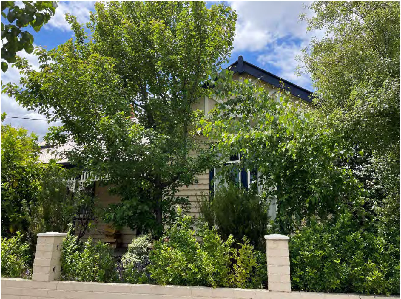
Figure 1. 230 Jasper Road, McKinnon (GJM Heritage, December 2022).
