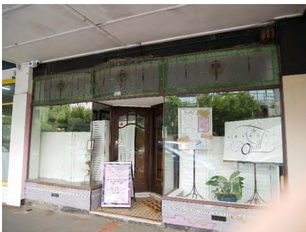
Figure 15. Shopfront at 141 McKinnon Road (GJM Heritage, February 2023).
