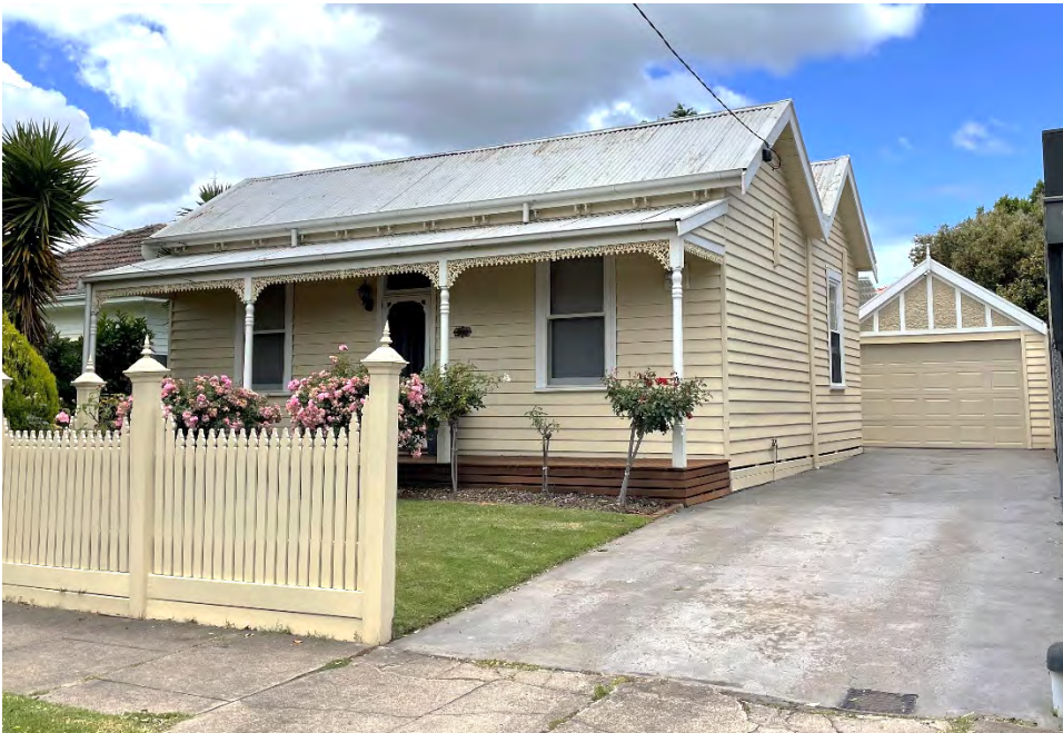
Figure 4. The north and west elevations (GJM Heritage, December 2022).
