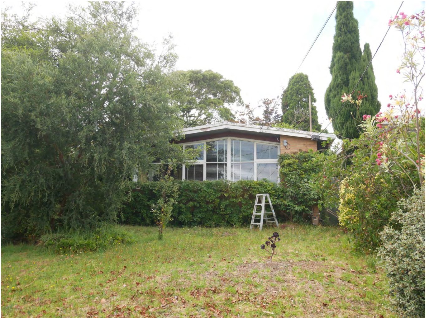
Figure 1. 18 Clee Street, McKinnon (GJM Heritage, February 2023)
