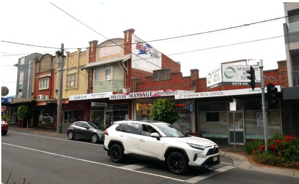
Figure 14. Looking south-east at 146-154 McKinnon Road (GJM Heritage, February 2023).
