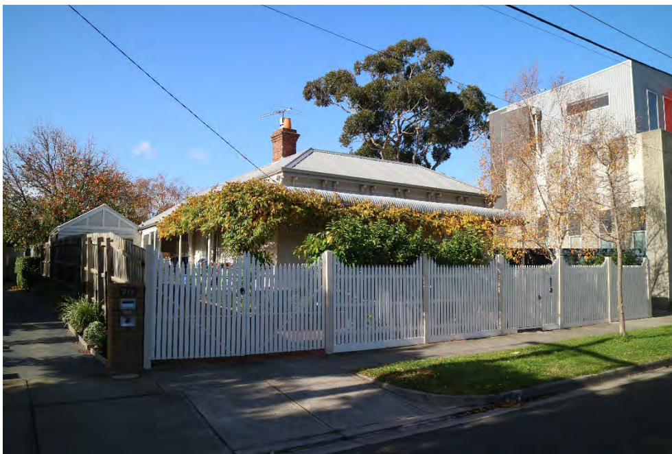
Figure 6. The principal (west) elevation and side (north) elevation (GJM Heritage, May 2023).
