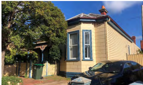
Figure 7. 9 Vickery Street, Bentleigh (Source: GJM Heritage, May 2022)
