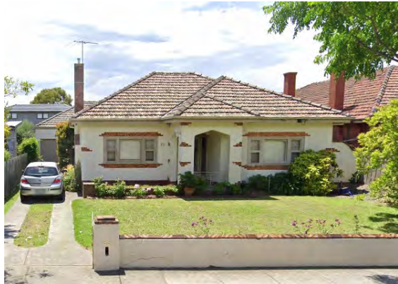
Figure 26. 29 Field Street, McKinnon (Source: Google Street View)
