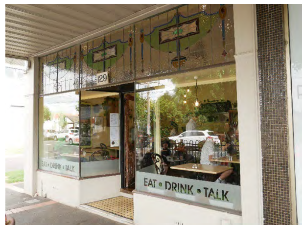
Figure 16. Shopfront at 129 McKinnon Road (GJM Heritage, February 2023).
