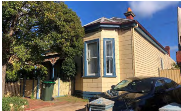
Figure 8. 9 Vickery Street, Bentleigh (Source: GJM Heritage, May 2022)
