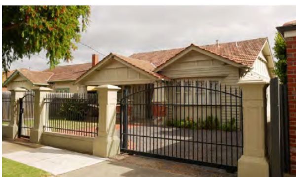
Figure 9. 37 Field Street, McKinnon (Source: GJM Heritage, December 2022)
