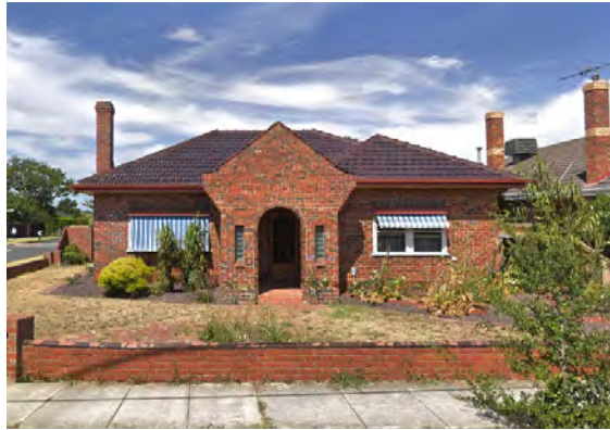
Figure 20. 22 The Highway, Bentleigh (Source: Google Street View)
