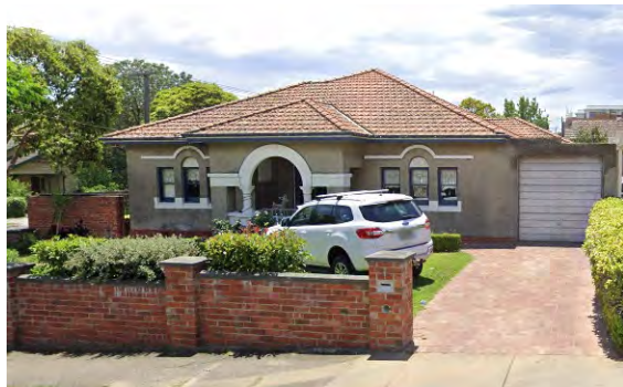
Figure 25. 1 Field Street, McKinnon (Source: Google Street View)
