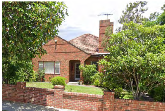
Figure 27. 22 Field Street, McKinnon (Source: Google Street View)
