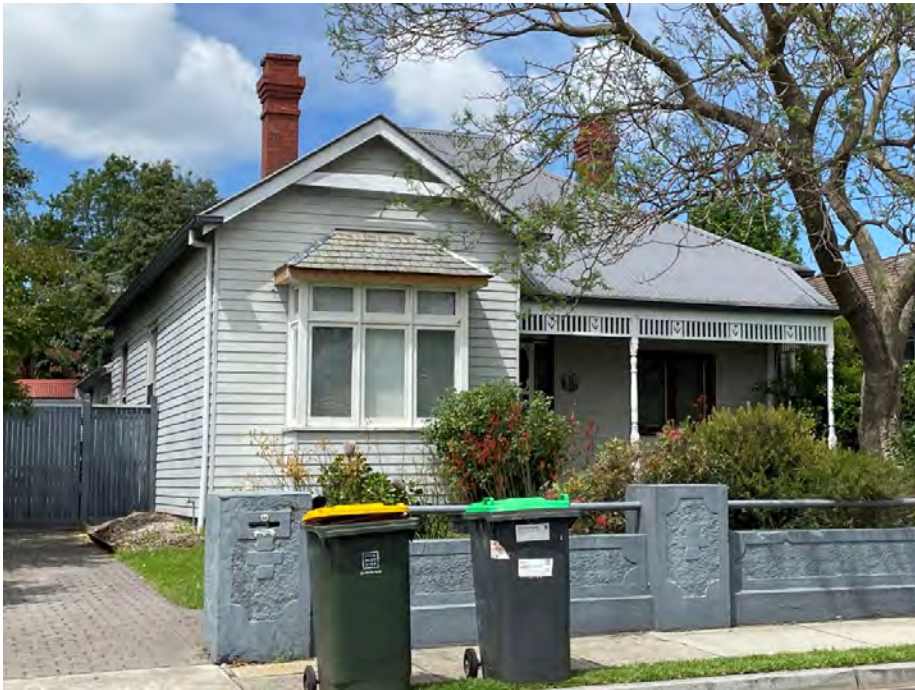
Figure 6. The north and east elevations (GJM Heritage, December 2022).
