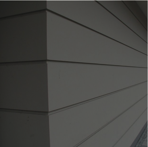
JAMES HARDIE STRIA CLADDING: DARK GREY PAINT FINISH
