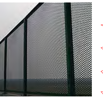
WELDMESH SCREEN/ FENCE - DARK GREY POWDERCOAT FINISH
