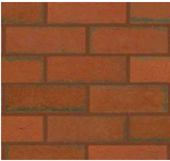
STRETCHER BOND BRICKWORK: BURWOOD BLUE FINISH
