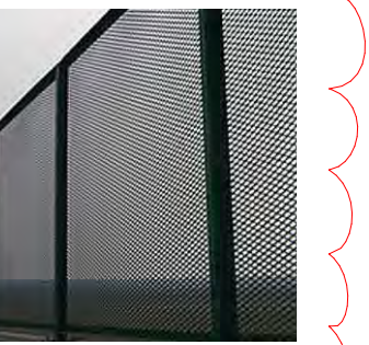
WELDMESH SCREEN/ FENCE - DARK GREY POWDERCOAT FINISH
