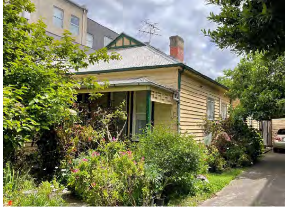
Figure 18. 123 McKinnon Road, McKinnon (Source: GJM Heritage, McKinnon Heritage Review, 2023)
