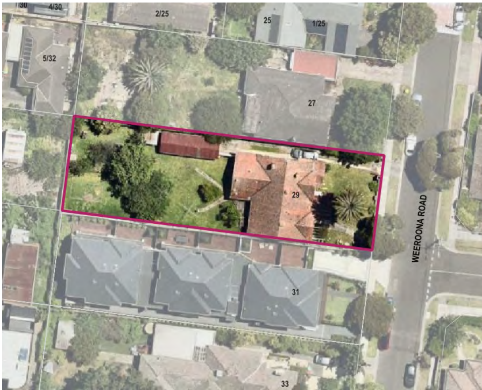
Figure 16. Recommended Extent of Heritage Overlay
