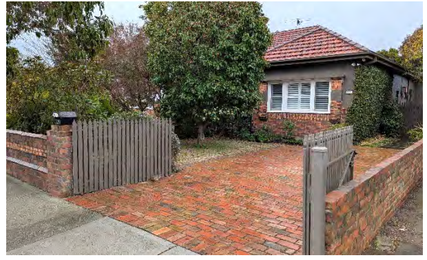
Figure 10. 320 Koornang Road, Carnegie (Source: GJM Heritage, September 2025)
