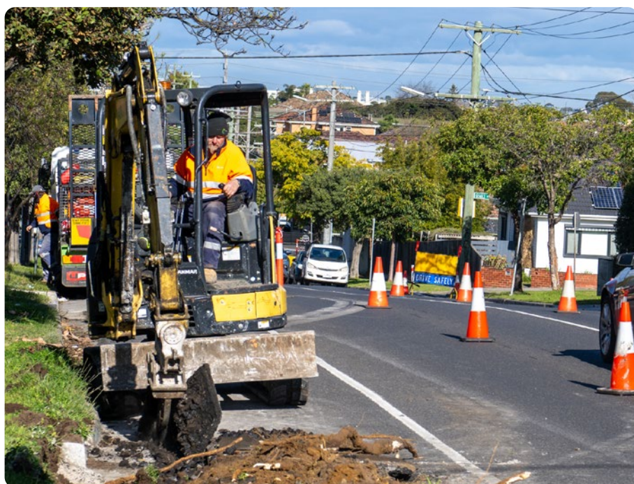
Kerb and channel renewal works improve the condition and safety of local streets across Glen Eira.
