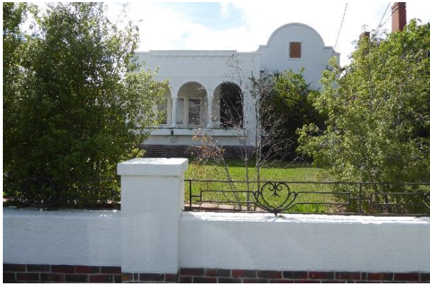
3 Shoobra Road Spanish Mission style frontage with barley twist columns to arched porch, render walls and parapet largely concealing Victorian period chimney, 1930s fence
