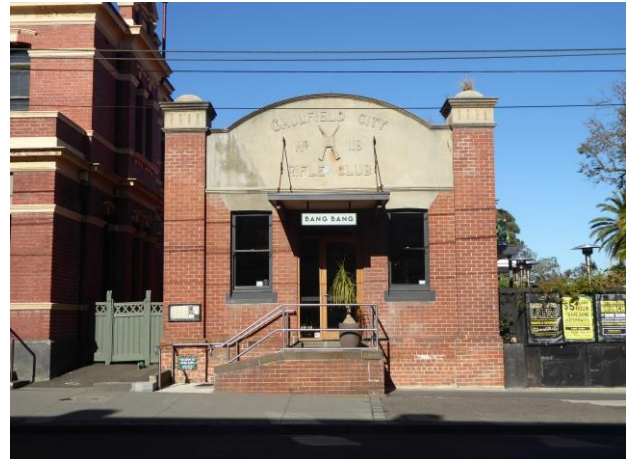
294 Glenhuntly Road – former Elsternwick rifle club, built 1915 Red brick and render, broad piers surmounted by domes, original entrance canopy, basalt sills
