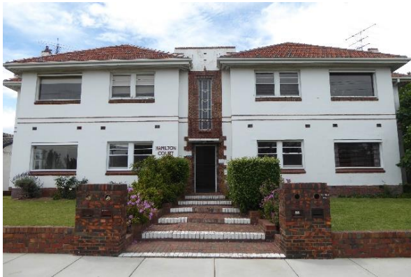
14 Orrong Road, Hamilton Court Moderne style influence to these flats, rendered with tapestry brick to entry and piers of original low brick fence, steel-framed stairwell window with chevron motif
