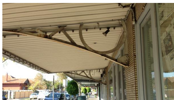
Original metal brackets to awning
