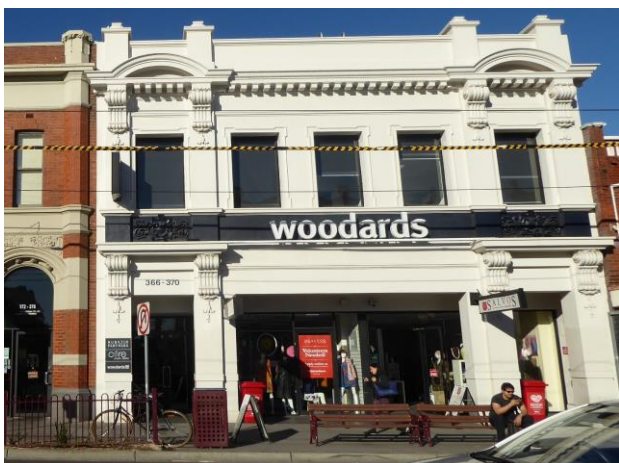
366-370 Glenhuntly Road National Bank, built 1915 Academic classical, prominent dentiltated cornice, plain parapet, end bays with curved pediments and console brackets
