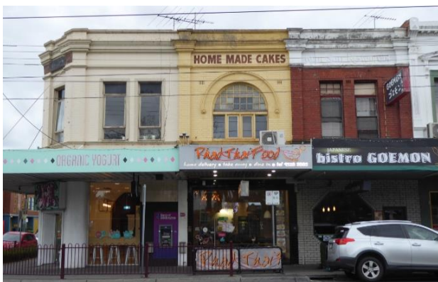
277-281 Glenhuntly, built 1902/03 (no. 277 possibly constructed a few years later); a group of three at corner of Selwyn Street, Red brick and render (overpainted to nos 277-279) Relatively plain cornice and parapet; central semi-circular arched window, multi-paned toplights (many replaced), also at no. 315
