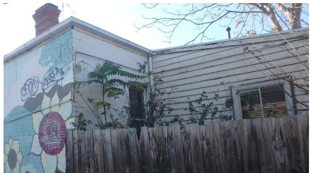
Intersection of brick and rear timber sections
