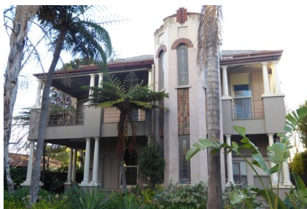
No. 16/ Ottawa – Note to tower-like bay: variegated face and tapestry brick voussoirs, panels and keystone, and lancet windows with clear/ripple glass/leadlighting combination
