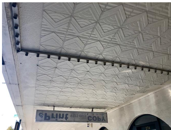
Original pressed metal soffit to awning with chevrons
