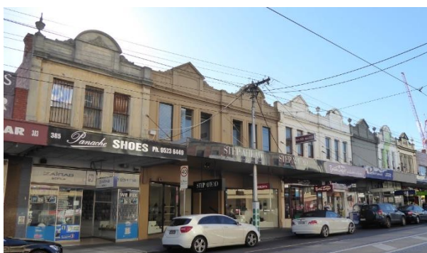
385-399 + 405 + 409 Glenhuntly Road Originally a group of 13 (built 1890), 3 of which have been modified/replaced Triple windows, parapet with some urns surviving and alternating triangular and arched pediments
