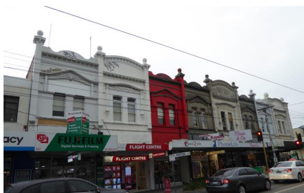
357-371 Glenhuntly Road Buckridge's Buildings, 8 premises built in two stages – 1911 (eastern four) and 1914 (western four) Parapet with scalloped sections and orbs Render finish remains unpainted to nos 363 and 367 Sinuous floral decoration (Art Nouveau style) above paired windows, framed by thin fluted pilasters
