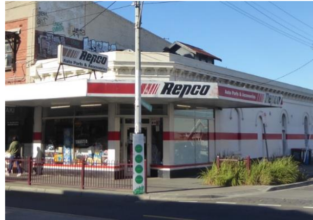
466-468, built circa 1889 Single-storey with visible lantern; ornate cornice, presumably items removed from parapet; arched openings and niches to side elevation; and canopy soffit with pressed metal
