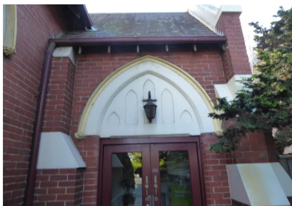
East side, entry porch. Tympanum with lancets in bas-relief, string moulding terminating with a boss
