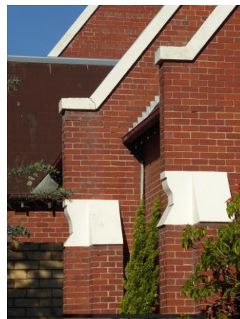
North elevations – curved corbels
