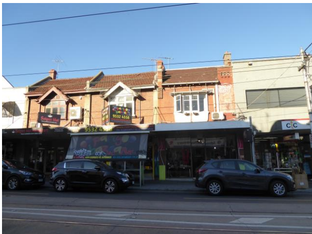
350-352 and 354-356 Glenhuntly Road, all built 1913 Tiled roofs, chimneys, red brick and render nos 350-352 – roof of 350 survives behind modified façade, red brick, brown brick toplights, slate roof nos 354-356 – gable window with casements, rendered piers
