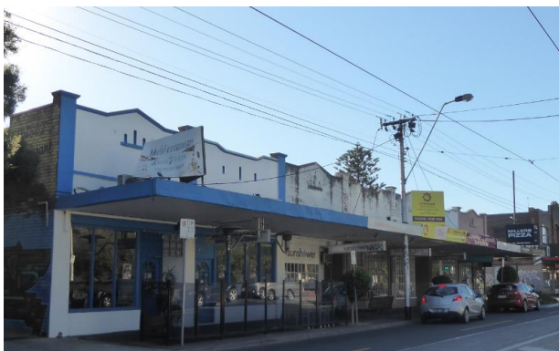
515-523 Glenhuntly Road Row of 7, built early 1920s Rendered parapet with alternating profile, separated into bays by plain piers
