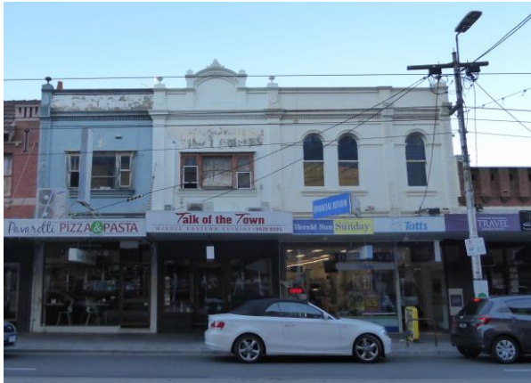
444-448 Glenhuntly Road Arched windows (altered to nos 446-448) Pilasters with fluting or vermiculation Remnant urns to parapet
