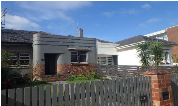
71, 71A, 71B Shoobra Road Unusual co-joined group of three, Moderne style, curved central bay, rendered with speed lines, brick plinth and window trim, possibly concrete tiles
