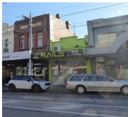
315 + 317 Glenhuntly Road No. 315 – red brick with rendered decorative elements (sills, panels, string mouldings, etc.), long windows with casements and toplights, visible chimneys; No. 317 – single-storey, rendered parapet with cornice, orbs or the like probably removed from end piers
