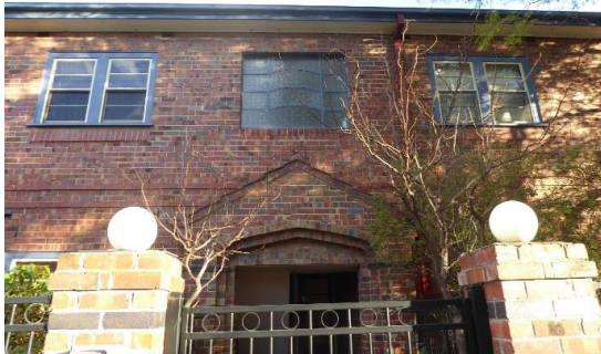
Gladstone Court Flats – steel-framed window with textured glass and bowed glazing bars
