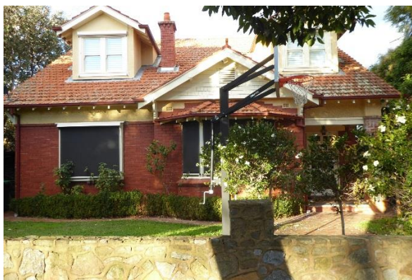
No. 19 – note exposed rafter ends, roughcast render banding and timber shingles and ventilator to the central gable
