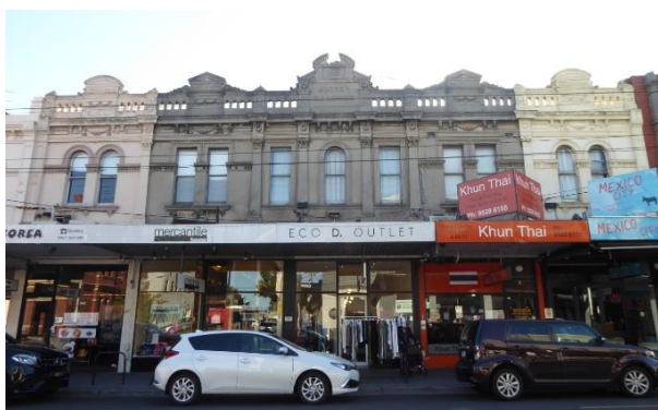
305-313 Glenhuntly Road Moore's Buildings, built 1891 Alternating arched and rectangular windows Cornice with festoons, wreaths, rosettes and brackets Pediment with arched openings and elaborate plates
