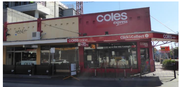
463-467 Glenhuntly Road 3 premises, originally part of a group of 5 Brick piers (overpainted) divide the wide rendered parapet Original steel-bracket at return of canopy.
