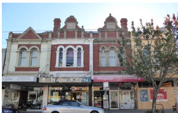
323-329 Glenhuntly Road Built 1889, T B Jackson architect Anglo-Dutch style, arched windows (some tripartite), tuck-pointed red brick and render (partly overpainted), (part) fluted pilasters, banded chimneys and partly visible roof
