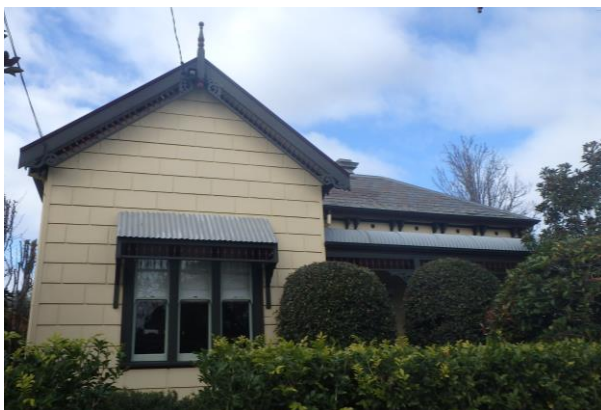
65 Downshire Road, Merrivale – asymmetric, ashlar boards, gable with three double-hung sash windows, slate clad roof. Bargeboard, frieze to verandah and hood with same design.
