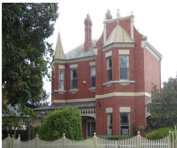
No. 32/34, Kenly – distinctive corner bay with lead lined pinnacle roof and cast iron cresting, timber verandah, and margin windows
