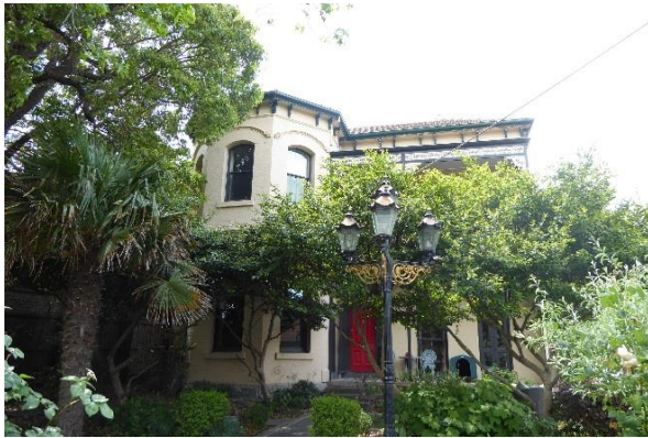
10 Orrong Road, Ascog 1887, Italianate style, two-storey, painted brick, arched windows with floriated mouldings, offset verandah with cast iron detailing linked to a non-original stair to south side.
