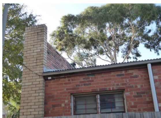
West elevation, north end Outer red brick skin of façade evident
