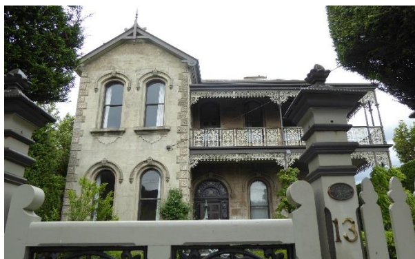
No. 13 –arched windows with Queen Anne sills and panelled door with sidelights and fanlight (leadlighting)
