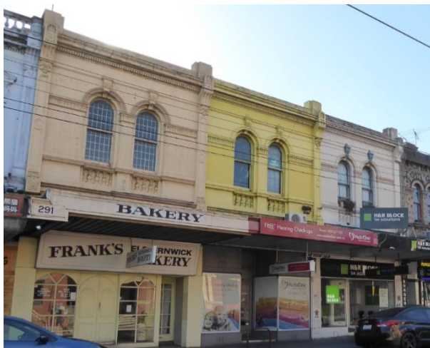
291-295 Glenhuntly Road – group of 3 Paired arched windows with bottled balustrade below, floriated band and dentillated cornice Balustrading and central plate to parapet removed, though evident in a historic image
