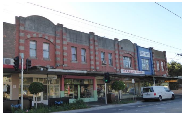
527-537 Glenhuntly Road Row of 6, built circa 1920 Red brick and render, with striped recessed arches and pilasters, Only no. 535 overpainted, and a large window replacing the paired format in the other premises; intact shopfronts to nos 527-531
