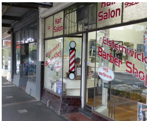
531 Glenhuntly Road – brown tiles to battered stall board, central recessed entry tiled, decorative glass screen over entry; nos 527-529 (background) are partly intact
