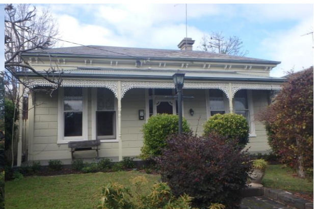
67 Downshire Road, Merleswood Symmetric façade, ashlar boards, paired double-hung sash windows, slate clad roof
