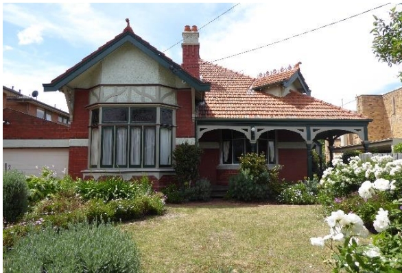
2 Orrong Road Queen Anne style with corner accent to roof, band consists of outer course of brown bricks and central roughcast rendered band, wide faceted bay window with decorative glass to toplights
