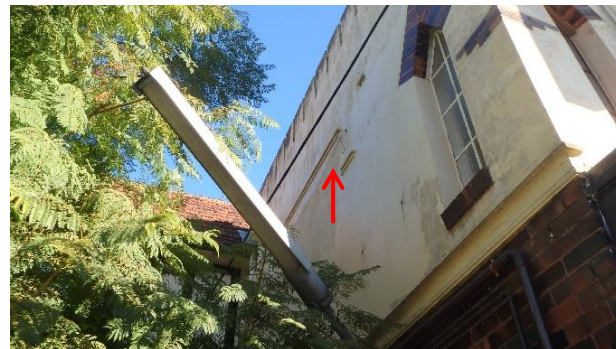
Lancet window and label moulding (indicated), east side of tower
