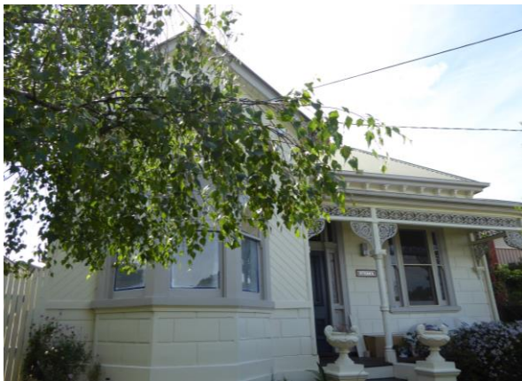
19 Shoobra Road Varied timber cladding – mainly ashlar boards with diagonal panelling to faceted bay, elaborate with keystones, distinctive cast iron verandah elements.
