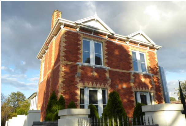
No. 15/Hartington – decorative semi-engaged column to windows
