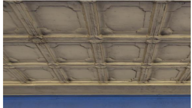
no. 377-381 Detail of pressed metal to canopy soffit
