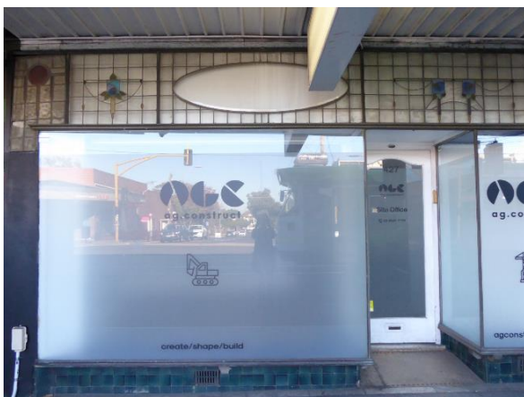
427 Glenhuntly Road – blue tiles to recessed stallboard, recessed tiled entry, and decorative glass to toplights.
