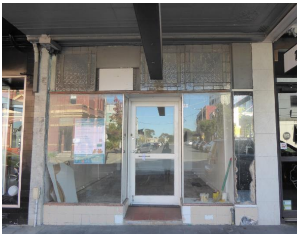
293-295 + 303 Glenhuntly Road (pictured) – copper finish, fine columns, glass with geometric configuration (visible to no. 293, probably obscured at no. 295), central entry with timber-framed door, frame to no. 305-307
