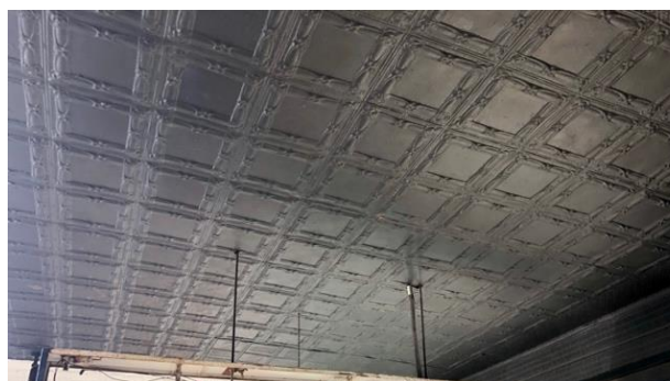
250 Glen Eira Road – pressed metal soffit
