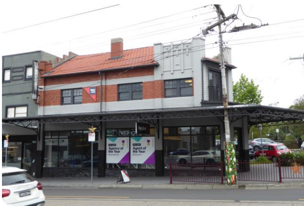
263 Glenhuntly Road, built 1918 Partial parapet and expressed roof, multi-paned upper sashes, rendered bands, decoration to rendered parapet sections, original steel-framed canopy with large brackets
