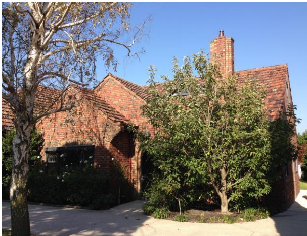
292 Glen Eira Road – clinker brick residence distinguished by its picturesque asymmetry, steeply pitched gables, corbelled eaves and herringbone brickwork panel (front gable)
