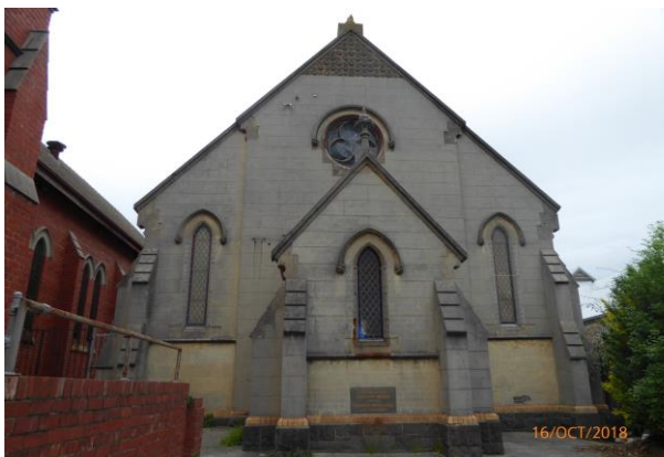
66 Orrong Road Initially Wesleyan Church, identified as Methodist from about 1905, later Uniting Victorian Period, 1887, designed by T J Crouch and built by Ireland & Newton for nearly £580. 2 Gothic style, rendered though initially bi-chromatic (a course of cream bricks are evident above the basalt plinth). Later employed as a school hall
