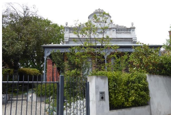
78 Riddell Street, Coolara Ornate rendered parapet with nameplate, bottled balustrade, urns and festoon. Bi-chrome brick to façade with quoining. Verandah to three sides.
