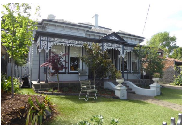
63 Shoobra Road, Wymswold Symmetrical façade, clad in ashlar boards, paired bays, slate clad roof, central pediment to verandah
