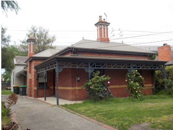
Photographs by Built Heritage Pty Ltd, October 2019
