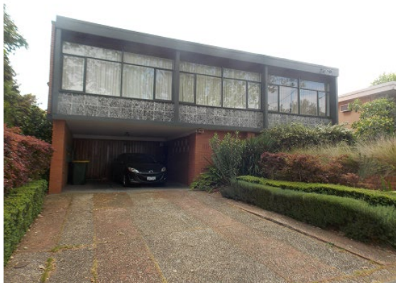
Photographs by Built Heritage Pty Ltd, October 2019
