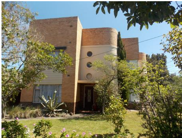
Photographs by Built Heritage Pty Ltd, October 2019
