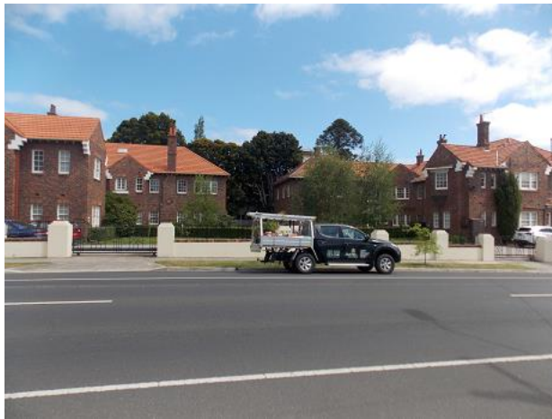
Photograph by Built Heritage Pty Ltd, October 2019
