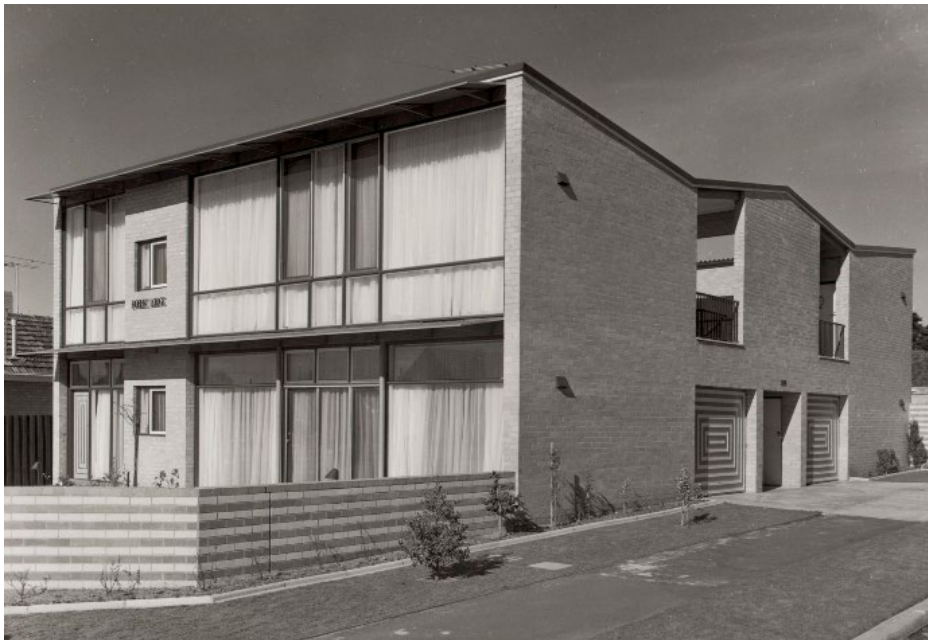
The virtually completed Robert Lodge , as photographed in 1959 by Wolfgang Sievers Source: Picture Collection, State Library of Victoria
