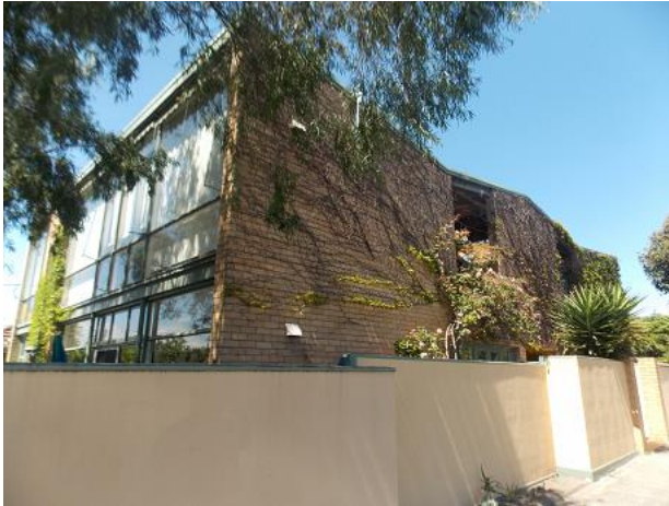
Photograph by Built Heritage Pty Ltd, October 2019
