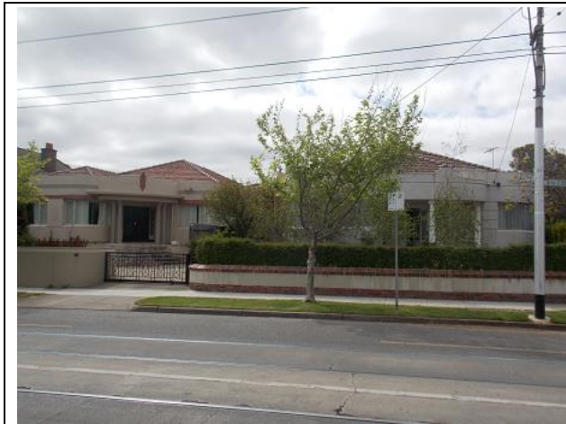
Photographs by Built Heritage Pty Ltd, October 2019
