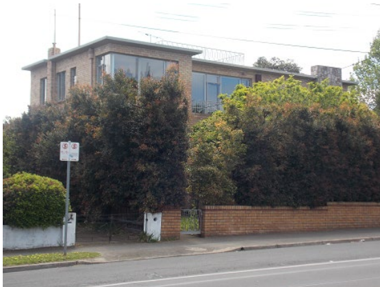
Photographs by Built Heritage Pty Ltd, October 2019
