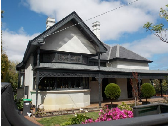
Photographs by Built Heritage Pty Ltd, October 2019
