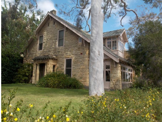
Photographs by Built Heritage Pty Ltd, October 2019
