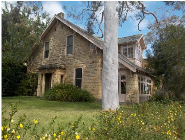
Photographs by Built Heritage Pty Ltd, October 2019
