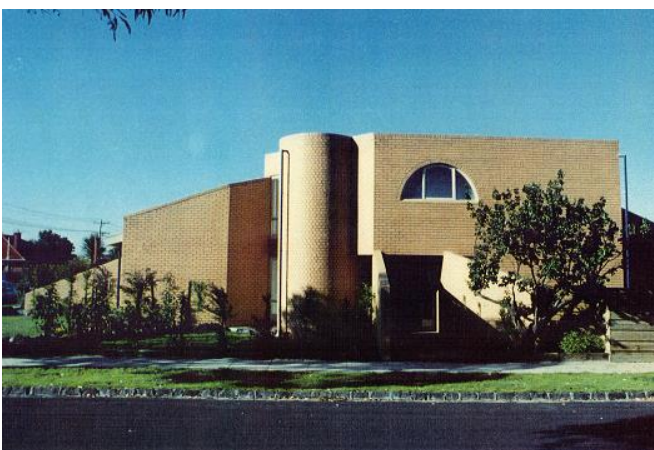
Contemporary view from the south (Goe Street) Source: courtesy Leon Fink, architect
