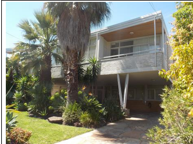
Photographs by Built Heritage Pty Ltd, October 2019
