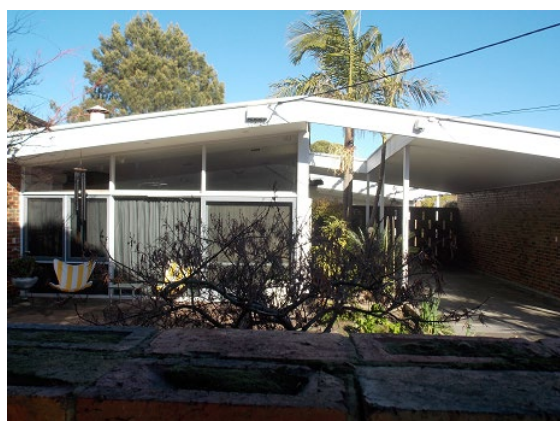
Photograph by Built Heritage Pty Ltd, October 2019
