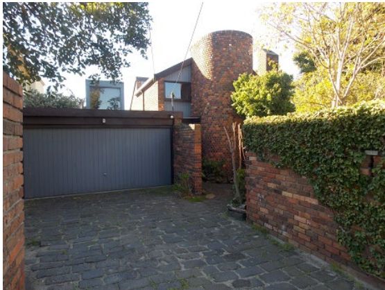
Photograph by Built Heritage Pty Ltd, June 2019
