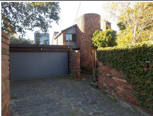
Photograph by Built Heritage Pty Ltd, June 2019
