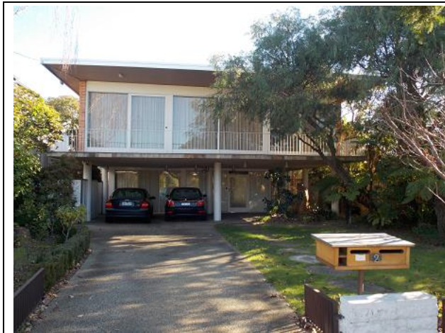
Photograph by Built Heritage Pty Ltd, June 2019
