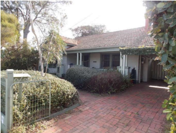
Timber bungalow at 13 Field Street (1925)
