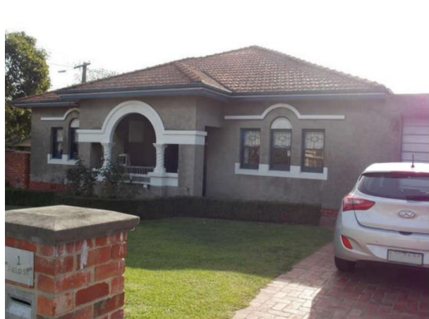
Rendered house at 1 Field Street (c1930)
