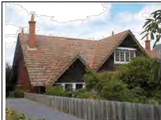
Photographs by Built Heritage Pty Ltd, October 2019
