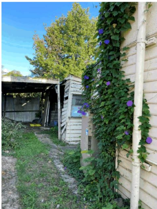
South-west of wall and rear carport with attached shed – Building wall not vertical, showing internal sub structure failure and rear carport and shed damaged beyond repair.
