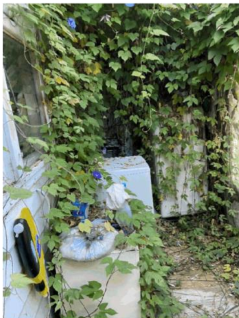
Inside of western extension – Roof calapsed and vegetation causing major structural decay.
