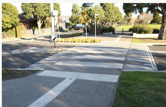
RAISED CROSSINGS: Raised crossings with the footpath ramped on a platform like a road hump, has been demonstrated to reduce crash rates and severity.
