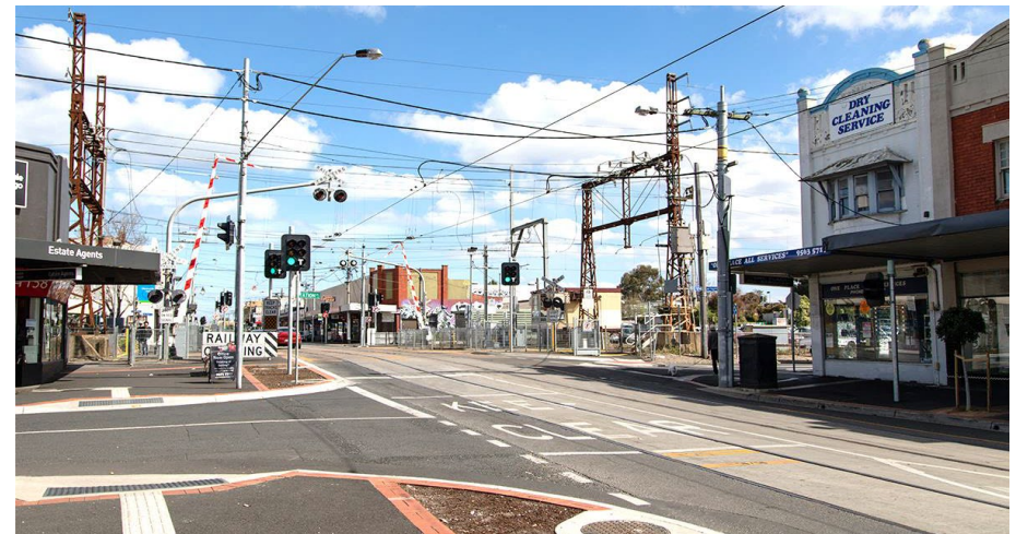
Glenhuntly Road Level Crossing (Images sourced from: State Government, Level Crossing Removal Project.)
