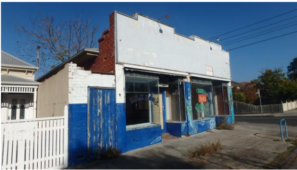
Façade – east end. NB infill section with timber door
