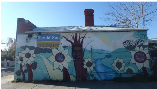
West elevation of brick section
