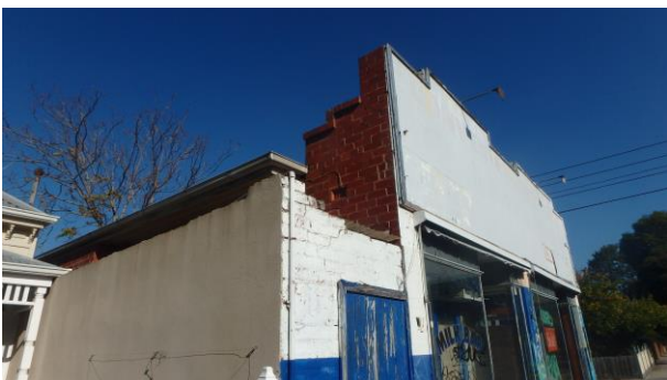
North-east corner Note setback of the hipped roof on the east side
