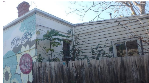
Intersection of brick and rear timber sections
