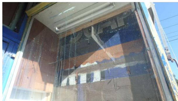
Signage to a likely original external wall Tuck-pointing evident
