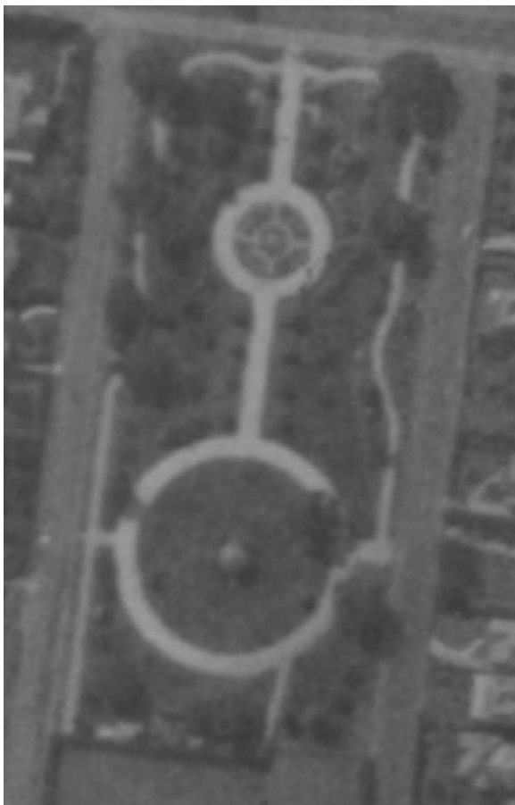
1931 aerial photograph of Hopetoun Gardens North is top of frame (Source: Landata, Maldon Prison , Run 24, Frame 2491)
