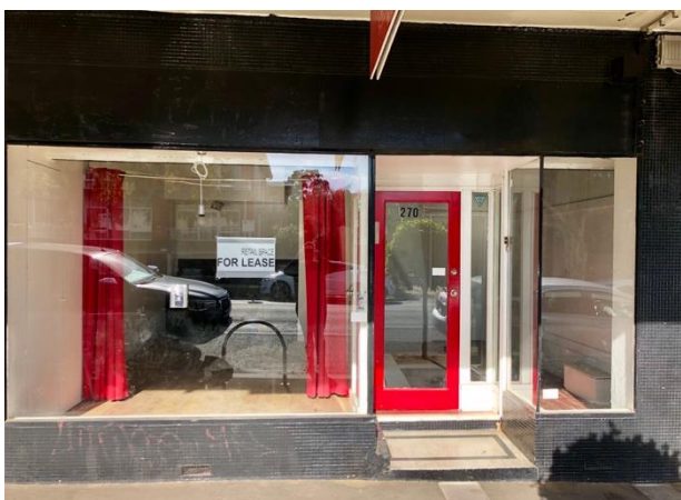
270 Glen Eira Road – intact shopfront
