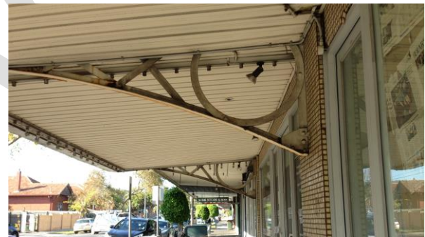
Original metal brackets to awning
