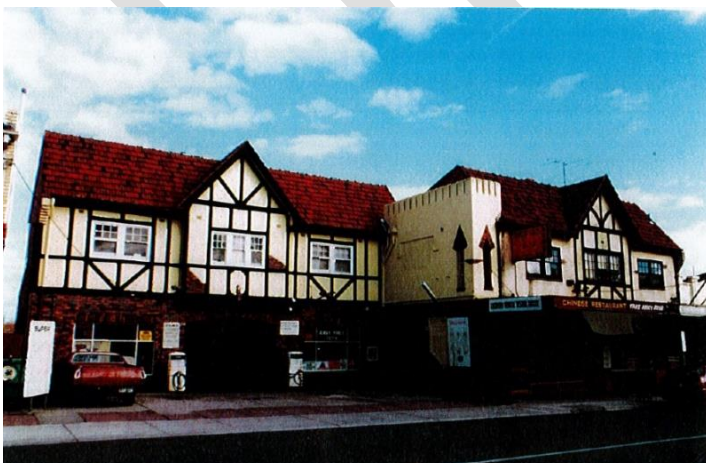
1997 photograph of E K Motors and shops. Note pumps have been repositioned (Source: Andrew Ward, City of Glen Eira Heritage Management Plan , 1997)
