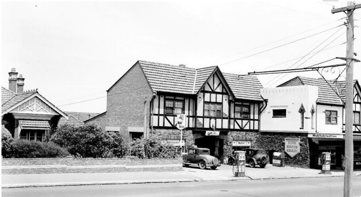
1954 photograph of Tudor Station , centre frame, and associated shops right of frame (Source: Laurie Richards Studio, ‘Garage at E/WICK’, January 1954, Museums Victoria Collections, item MM50717)
