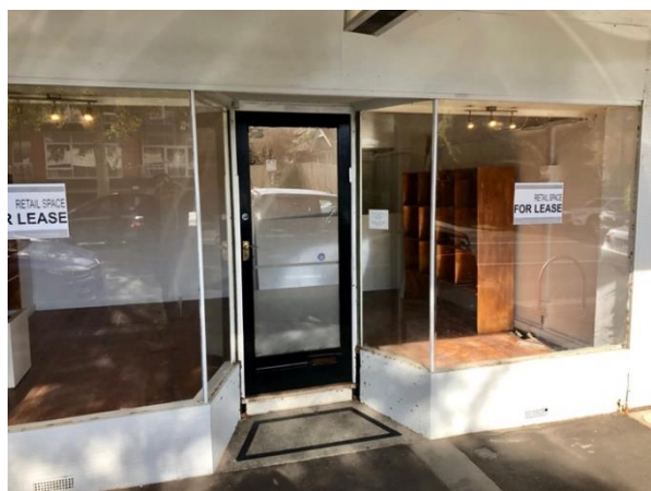
274 Glen Eira Road – intact shopfront
