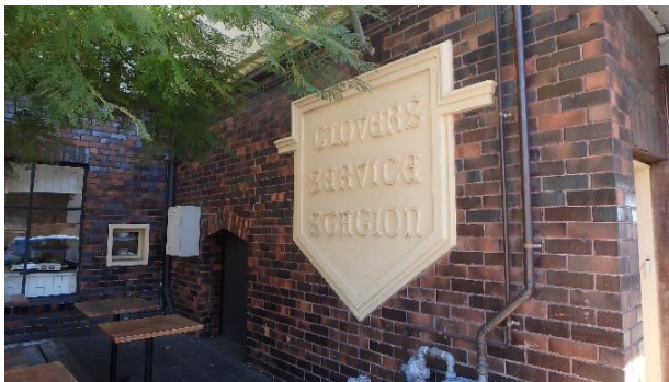
Sign, eastern side of tower
