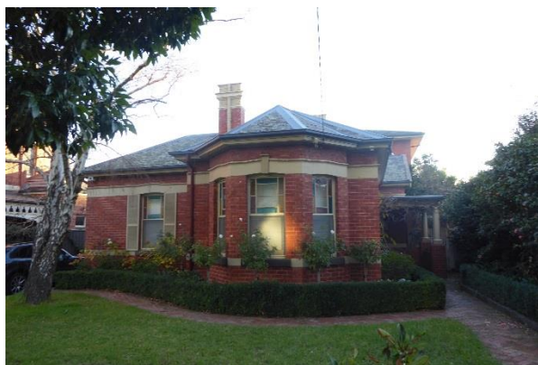
No. 30/ Maescourt – side porch with flat roof and Tuscan columns and margin windows (top panes only) with multicoloured glazing
