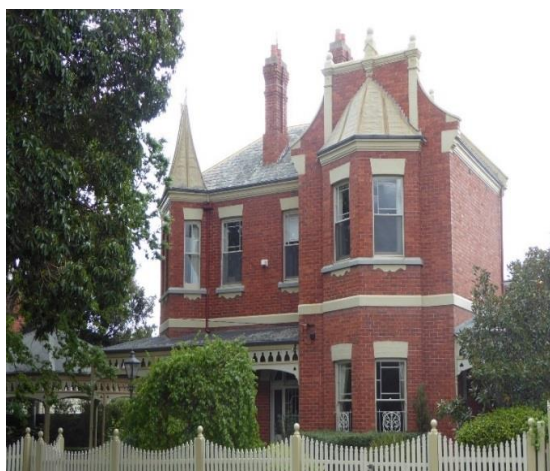
No. 32/34, Kenly – distinctive corner bay with lead lined pinnacle roof and cast iron cresting, timber verandah, and margin windows
