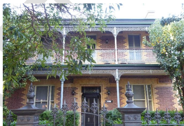
No. 12/ Monkleigh – label moulding and tapestry brick voussiers, ground floor
