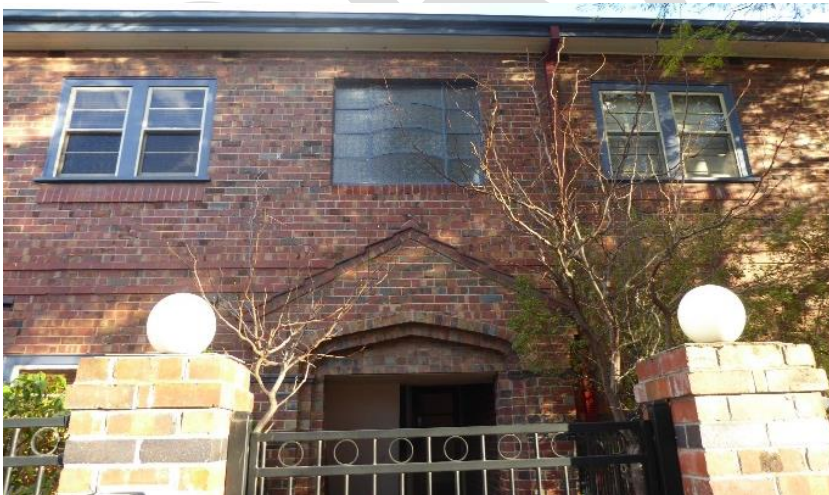
No. 7/Gladstone Court Flats – steel-framed window with textured glass and bowed glazing bars
