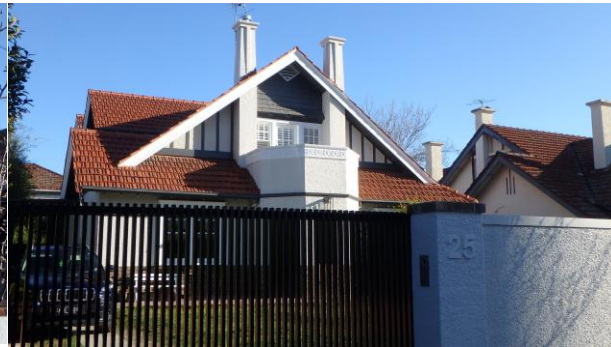
25 Stanley Street Arts and Crafts style, broad gable end with tapered chimneys piercing roof, floriated band to central balcony
