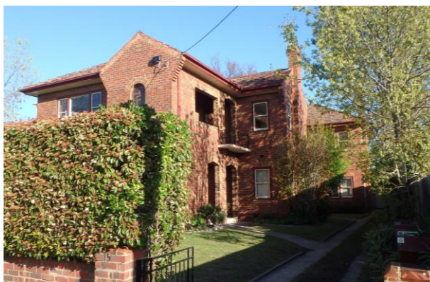
15 Stanley Street Durham Old English style, clinker brick with some tapestry bricks to openings, Tudor arches, original fence
