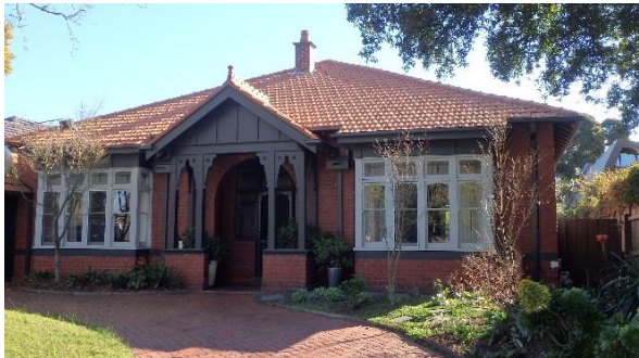
8 Victoria Street Symmetrical façade with distinctive porch with timber screen, arched entry opening, and recessed doorway
