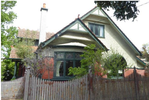
88 Shoorbra Road Arts and Crafts style, extensive use of roughcast render, tall tapered chimneys, constructed by local builder, Samuel Brook, during 1910-11
