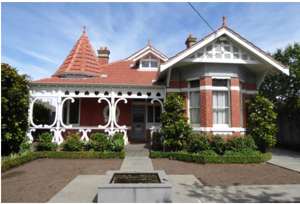
2 Shoobra Road Queen Anne style with corner conical roof, distinctive timber verandah with alternating heart frieze and large curvilinear members, decorative glass to entry and porthole window
