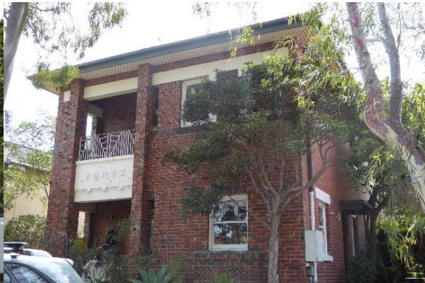
5 Shoobra Road, Boree Clinker brick flats with some Art Deco detailing, primarily the geometric pattern of the stained glass and metal balustrade, original fence
