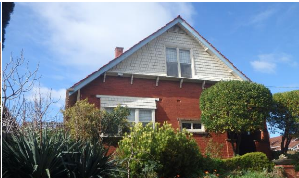
77 Shoobra Road Arts and Crafts style with attic, red brick and extensive use of shingles to skirt and roof to boxed-framed window
