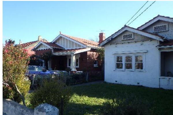
29, 35-51 Parkside Street, nos 41+ 43 Generally bungalows with gable roofs, with the ridges being either perpendicular or transverse (parallel) to the street
