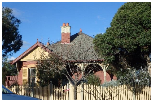
56 Orrong Road Built 1900 as a ten room house, 1 red brick with cream and brown brick banding, cream brick lintels, slate clad roof with pyramidal main section
