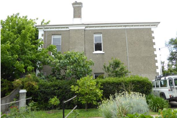
21 Elm Avenue Walton , 1886. Modified two storey mansion. Main elevation is to the west, obscured, with a masonry stair added. More intact to side and rear (along railway line). A roughcast render has been added though the quoining retains a smooth finish.
