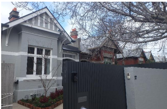
37-51 Downshire Road, no. 37 in foreground Group of similar paired, semi-detached cottages, chimneys with rendered caps and terracotta chimney pots, red brick with rendered band and lintels, remnant tuck pointing
