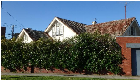
32 Riddell Street Two storey, distinctive Griffinesque window detail, located unusually high in wall, possibly (part) concrete walls
