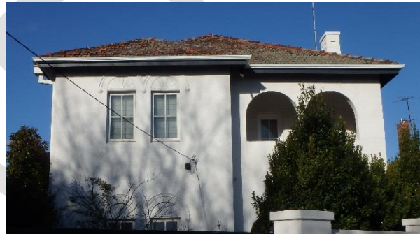
34 Riddell Street Mediterranean style, arched porch openings to both level, cartouche to ground floor, walls combination of smooth and roughcast render
