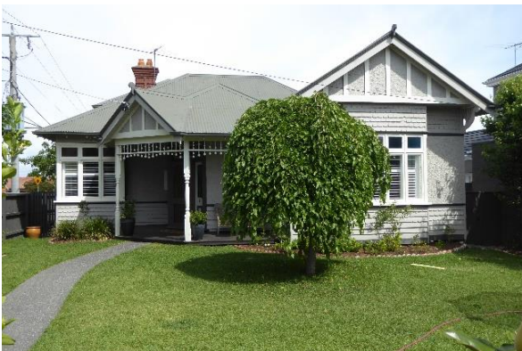
52 Shoobra Road Timber-framed with shingled boards and roughcast sheeting, corner verandah with spindle frieze
