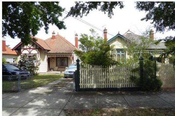
74-86 Shoobra Road, nos 74-76 pictured Group of similar weatherboard houses with consistent form, chimneys and gable end treatment
