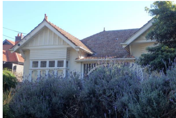
4 Victoria Street Symmetrical façade with paired gable ends with varying detailing and bays, timber-framed, porch with arched screen
