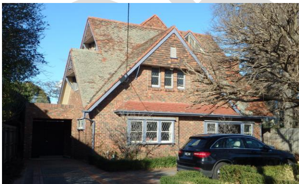
40 Riddell Street Old English/Tudor Revival style, terracotta shingle cladding to roof, Roman bricks to first floor window, diamond quarrels to window sashes
