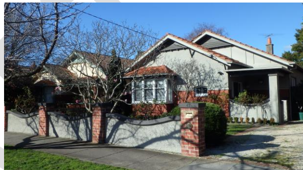
45+47 Victoria Street Bungalows with double street-facing gable ends with small shingled skirts, red brick and roughast render
