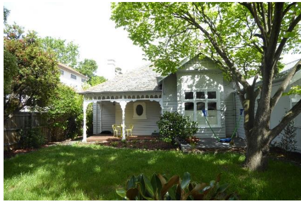
28-40 Shoobra Road, no. 34 pictured Group of brick and weatherboard Queen Anne style houses with bay windows
