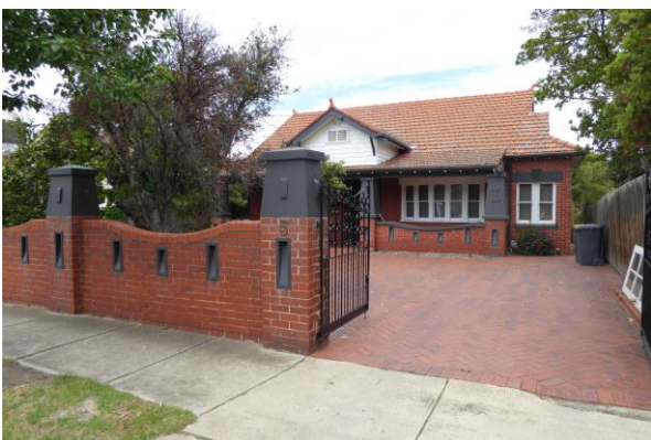
5 Stanley Street Bungalow style, roof with transverse ridge, porch with tapered piers, original fence
