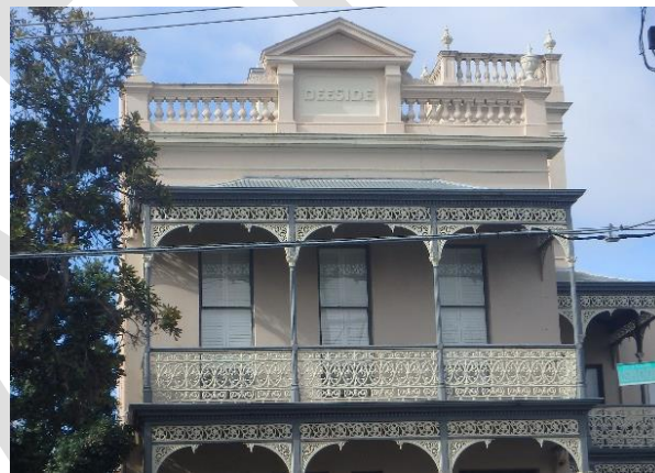
47 Shoobra Road, Deeside Italianate style with recessed tower, ornate parapet with pedimented nameplate and bottled balustrade surmounted by urns.
