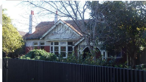
32 Victoria Street Arts and Crafts style with long transverse gable roof, extensive use of leadlight
