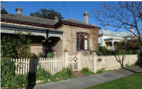
1-3/7-17 Gisborne Street (odds) & 15-23/29-35 (odds) Orrong Road Victorian villas with mostly consistent detailing including chimney caps and mouldings, main arched window in a projecting plane, some with label moulding. Some modified, four of 21 replaced. Some slate roofs remain.
