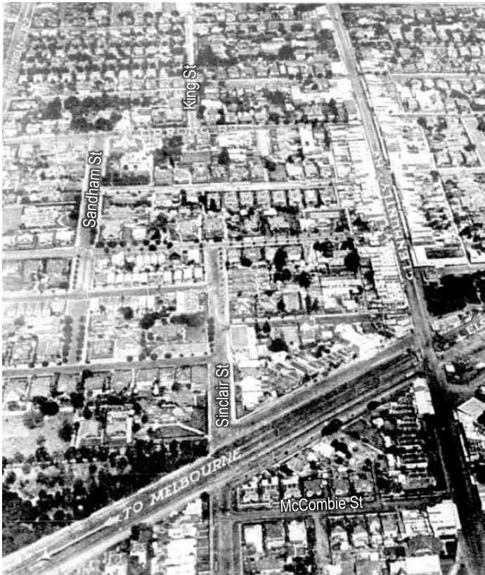
1926 oblique aerial photograph of the southern portion of the precinct (Source: 'Elsternwick from an Aeroplane', Weekly Times, 5 June 1926, p50)
