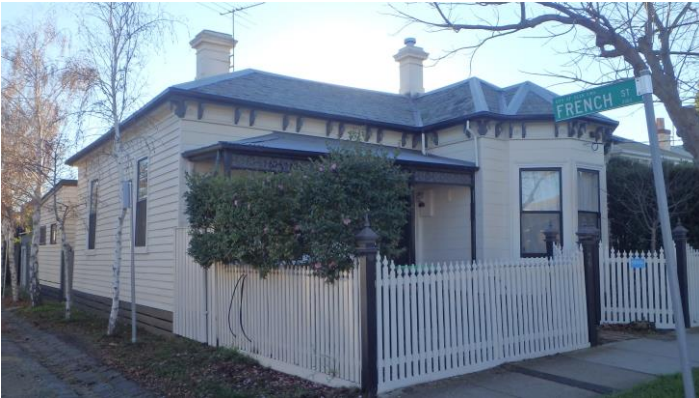
56 Regent Street Modest asymmetrical timber-framed Italianate villa, late Victorian period
