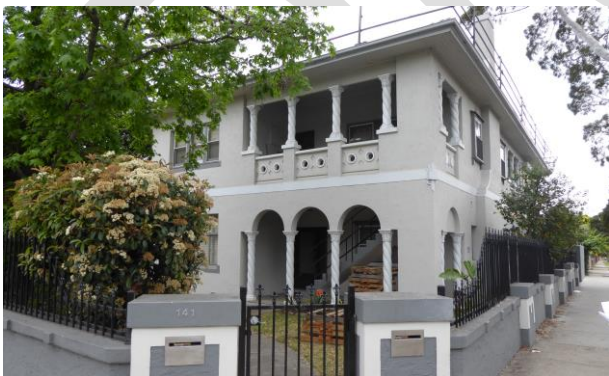
141 Orrong Road – triple arched loggia, elaborate balustrade and original fence
