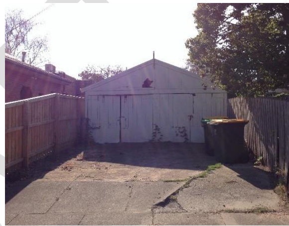
4 Garden Street – original/early rear shed or garage with timber folding door, viewed from Mulgrave Street.
