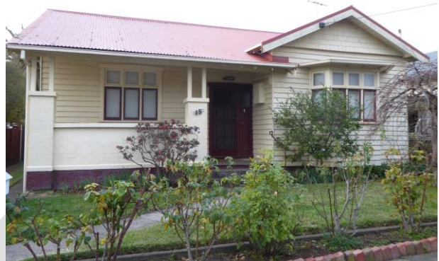
15 Prahran Grove – weatherboard with paired timber posts above masonry wall
