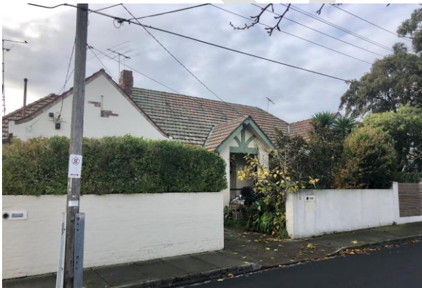
1 Mulgrave Street – distinctive elongated form with a façade defined by three street projecting gables, with half-timbering (curved bracing) to the central gable end and some tapestry brick banding
