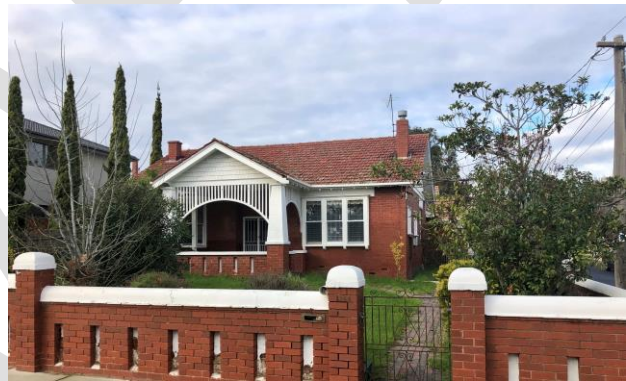
146 Orrong Road – prominent porch, tapered roughcast rendered piers and sinuous timber frieze (hint of Art Nouveau)
