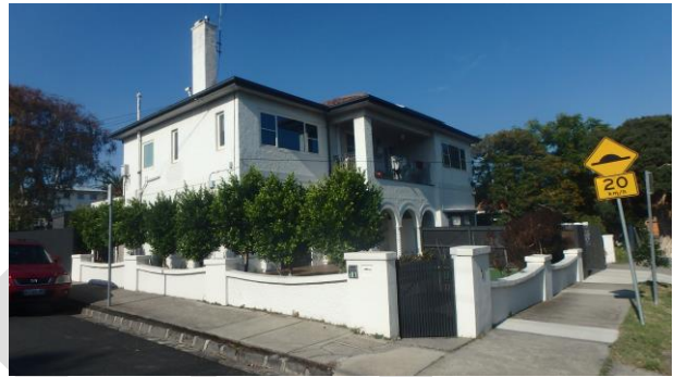
1-1A Somerset Street – textured render, triple arched loggia and bow window (with lead lighting)
