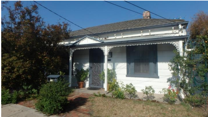
12 Mulgrave Street – bracketed cornice and cast iron frieze
