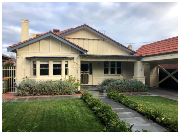
8 Prahran Grove – overpainted brick and rendered bungalow with faceted bay window and batted sheeting to the gable ends
