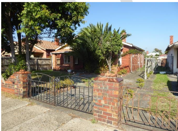
230 and 232 Glen Eira Road – clinker brick fence and metal gates
