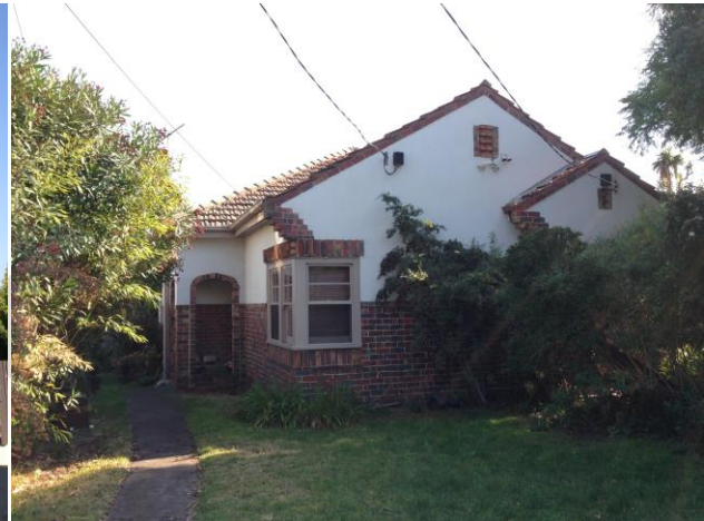
4 Garden Street – clinker brick contrasted with smooth render and Tudor arches to enclosed side porch
