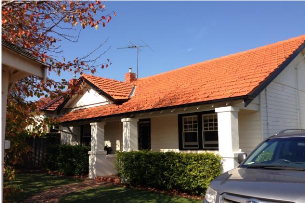
2 Mulgrave Street – weatherboard with brick balustrade and square piers in a roughcast finish
