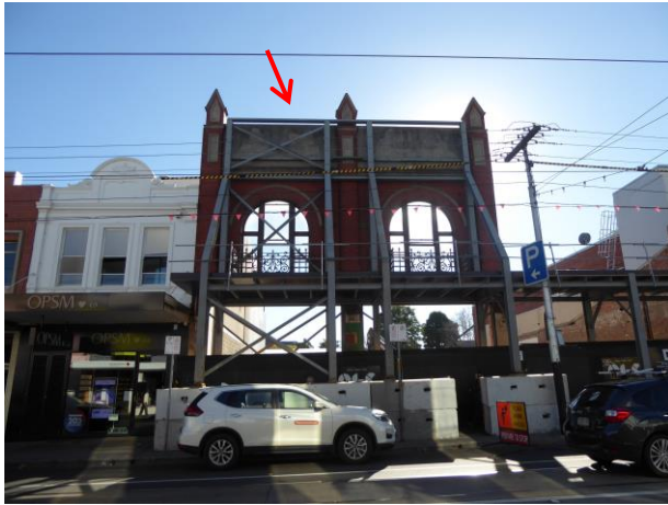
411-413 Glenhuntly Road (red arrow) Semi-circular arched windows with decorative balconette railing Parapet with gabled niches above the pilasters
