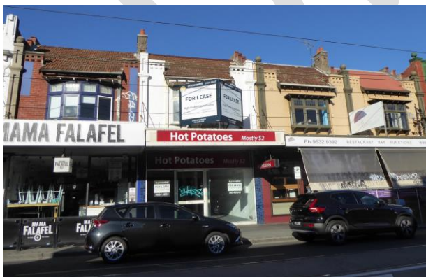
338-344 Glenhuntly Road, built 1913 Expressed roof with exposed rafter ends and chimneys, quarrels to toplights, red brick (overpainted to all but no. 344) nos 338-340 – box-framed windows nos 342-344 – curved, bay windows
