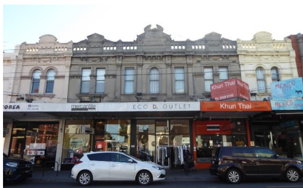
305-313 Glenhuntly Road Moore's Buildings, built 1891 Alternating arched and rectangular windows Cornice with festoons, wreaths, rosettes and brackets Pediment with arched openings and elaborate plates
