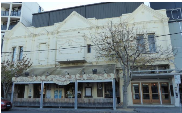
9 Gordon Street Built as hall in 1888, T B Jackson architect – prominent pediments, paired narrow windows, panelled or fluted pilasters Parapet has been modified (original profile evident in historic image)
