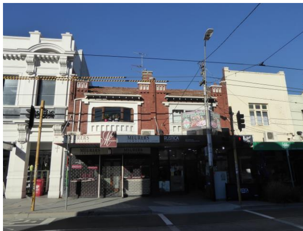
362-364 Glenhuntly Road (middle), built 1916 Tiled roof with exposed rafter ends, red brick, rendered central part and infilled balconies
