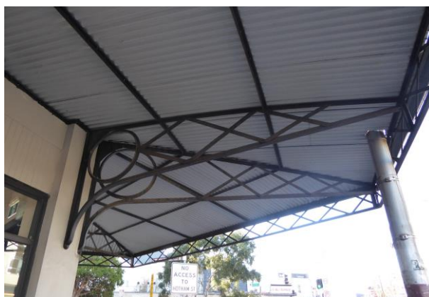
Canopy and bracket detail – no. 263 NB – original tramway pole
