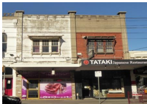
470-472 Glenhuntly Road Red brick and render (overpainted no. 472), boxed-frame window with multi-paned upper sashes, wide rendered frieze, piers
