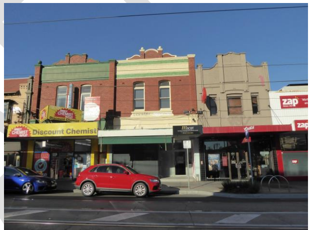
332 Glenhuntly Road (right) + no. 334-336 (left), no. 332 – built 1912, plain and roughcast render, brick (painted) piers; had been a pair with a rendered band and brickwork no. 334-336 – built 1913, red brick, wide frieze with original green tiles and roughcast render (obscured to no. 336), orbs to pediment
