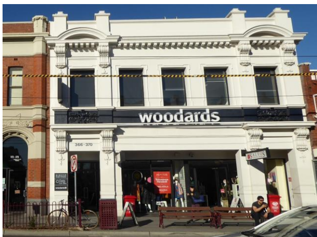
366-370 Glenhuntly Road National Bank, built 1915 Academic classical, prominent dentillated cornice, plain parapet, end bays with curved pediments and console brackets
