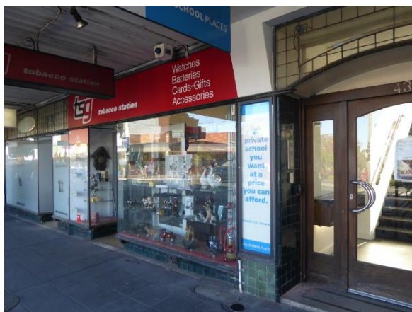
427 Glenhuntly Road (left) + no. 429 (middle) – blue tiles to recessed stallboards etc.; and no. 431 (right) – green tiles, timber door, granolithic step
