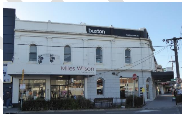
271 + 1 Gordon Street Fluted pilasters, arched windows, bas-relief panels, rusticated base to curved corner section Urns removed from parapet, evident in a historic image
