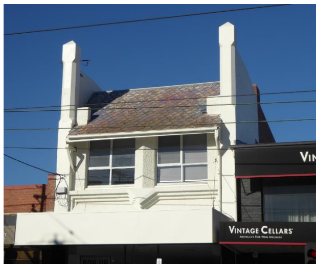
420 Glenhuntly Road Smooth and roughcast render, expressed roof clad in imbricated tiles/shingles (possibly terracotta), non-original windows
