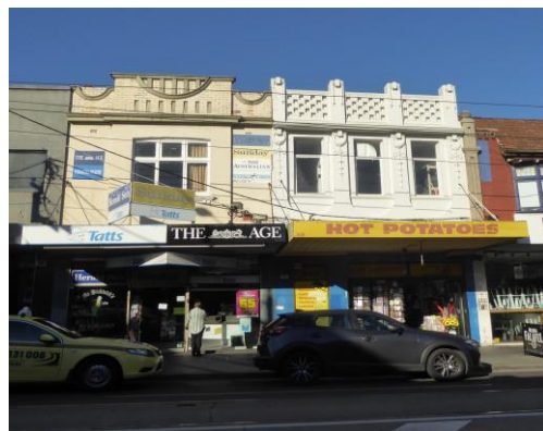
346 (right) + 348 (left) Glenhuntly Road, both built 1913 Both overpainted no. 346 – brick and render, 3 bays, wreaths and drop ornament to piers no. 348 – brick, scalloped parapet, casement windows
