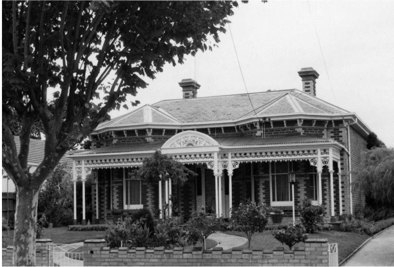
Late 1970s photograph of 51 Seymour Road – note mid-20 th century front fence (now altered) (Source: John T Collins, SLV, H95.200/1255)
