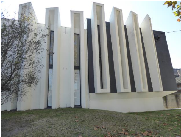
South façade – window hoods
