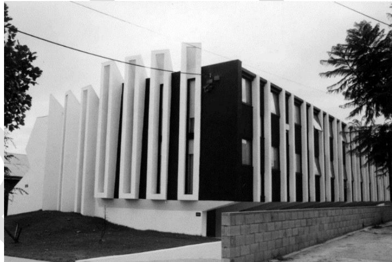
Townhouses photographed from Seymour Road in 1977 (Source: John T Collins, SLV, H95.200/1254)
