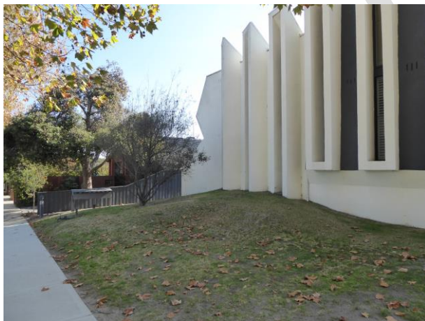
South façade – window hoods
