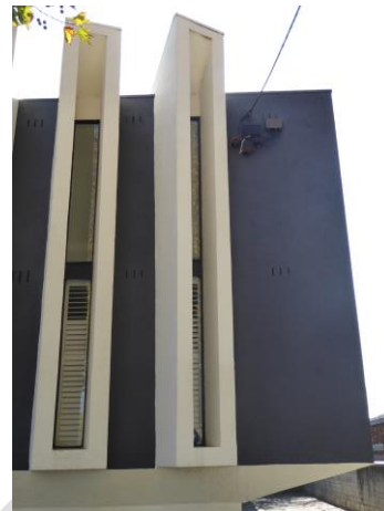
South façade - window hoods
