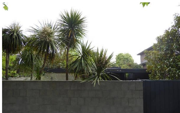
High wall to garage courtyard and view over flat roofs
