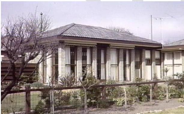
Photograph of the units (west façade) from Prahran Grove, late 1960s (Source: Peter Wille, SLV, H91.244/2047))
