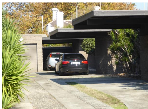
Cantilevered carports Driveway has been modified and the garage is a later addition
