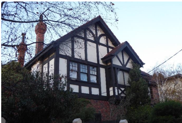
Façade, first floor, north end
