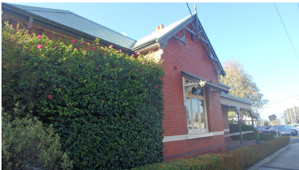
West elevation from Hotham Street
