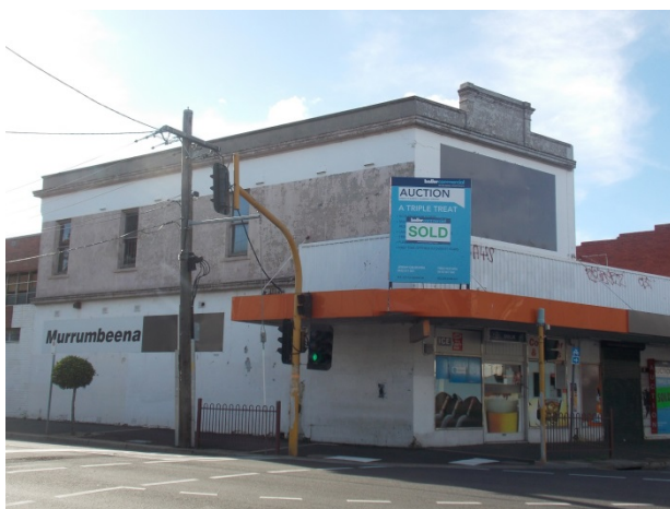
430-432 Neerim Road 2019 – south facing upper floor windows appear to be covered with signage hoarding. The identical pair to this shop has been demolished.
