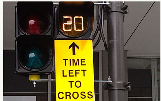
COUNTDOWN FOR PEDESTRIANS: Allows easier decision making when pedestrians approach intersections, or are crossing larger intersections.
