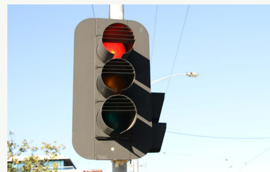
REST ON RED: Traffic signals sit on red until activated by a vehicle, while at all other times pedestrian signal sits on green.
