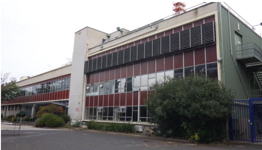
Exterior of Gordon Street Studios from car park. Photo by heritage ALLIANCE, 2018
