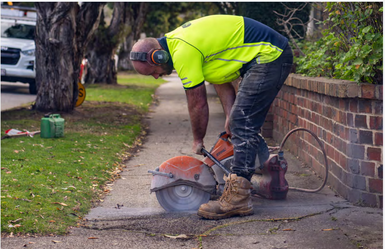
A contractor wearing personal protective equipment while conducting footpath repair works.
