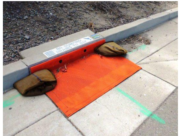
Figure 3 - Sediment Trap
