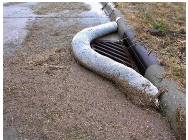
Figure 5 - Sediment Trap
