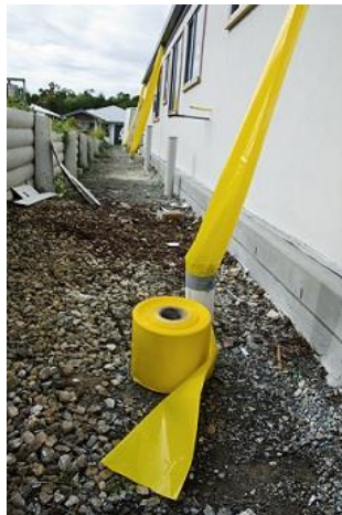
Figure 2 - Temporary Downpipes
